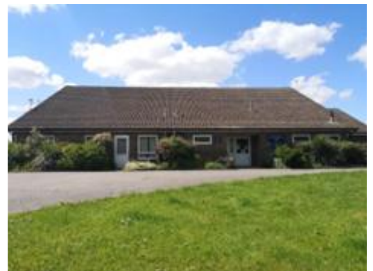
Kingswood Village Hall
