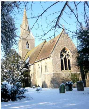
St Mary's Church Langley
