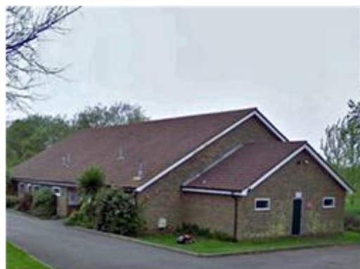
Kingswood Village Hall
