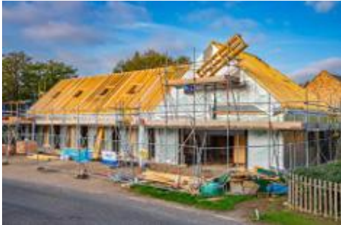
New village Hall under construction
