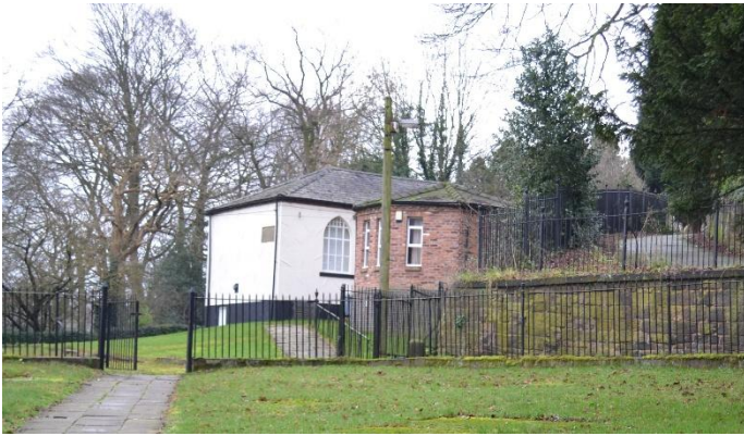
St. Peter's Parish Rooms exterior
