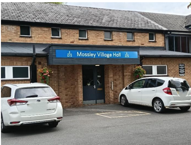
Mossley Village Hall exterior
