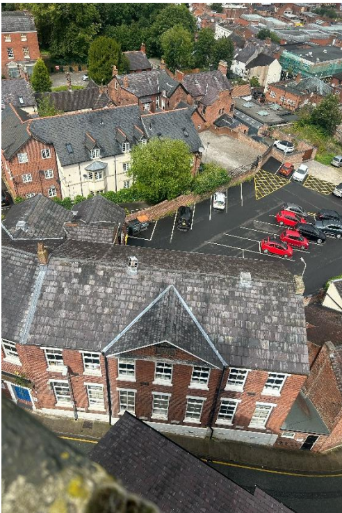
St. Peter's School exterior
