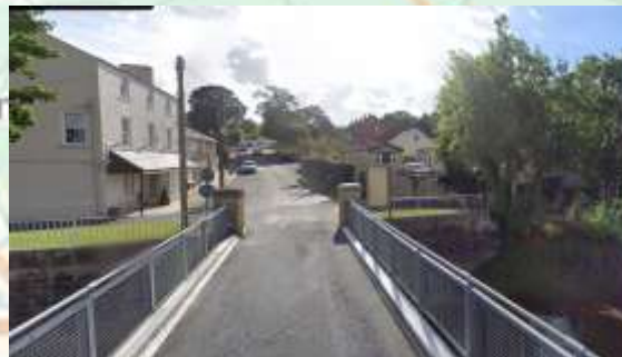
Cartford Bridge, Little Ecclestone
