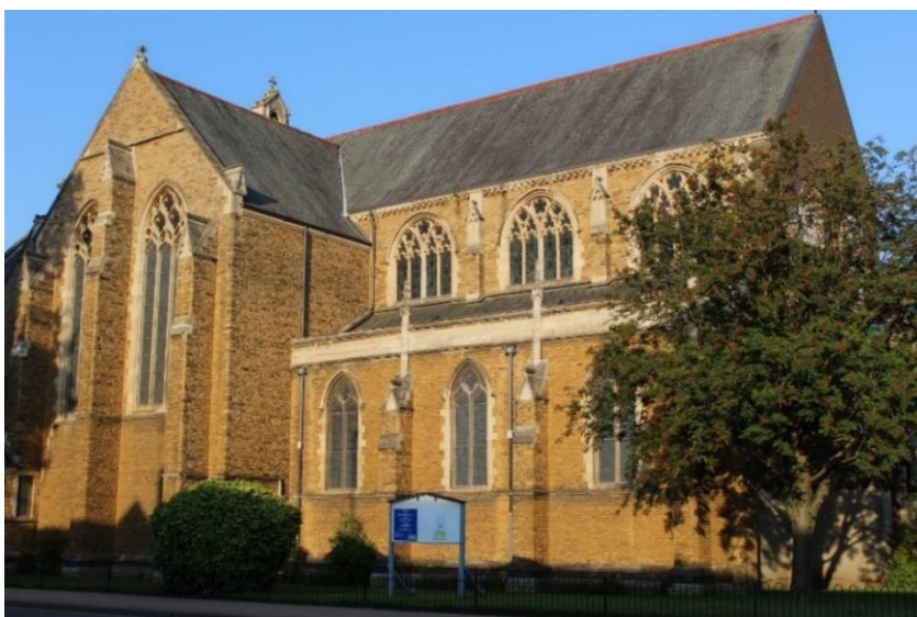
North elevation, fronting Wellingborough Road
