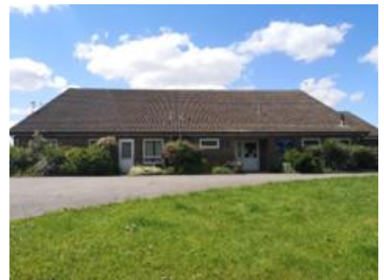
Kingswood Village Hall
