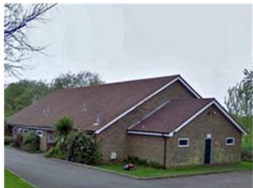
Kingswood Village Hall
