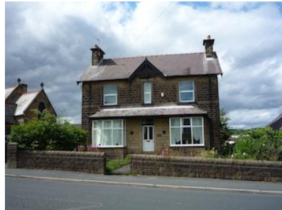
View of front of the house
