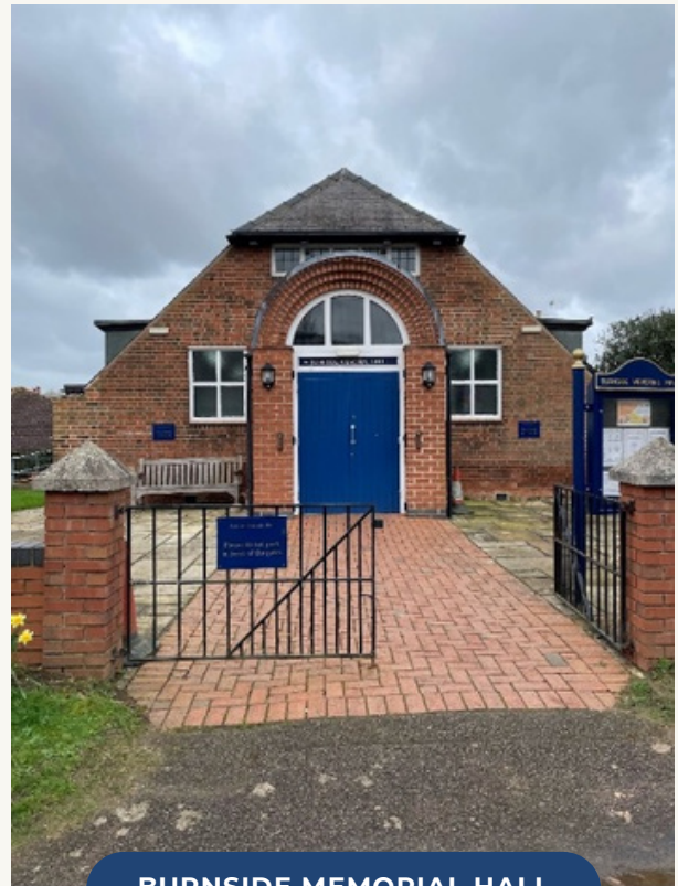
BURNSIDE MEMORIAL HALL
