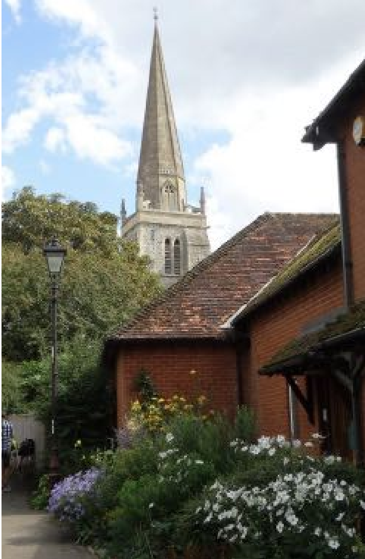
The Parish Centre building and front garden
