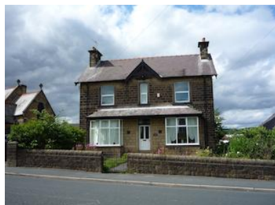
View of front of the house
