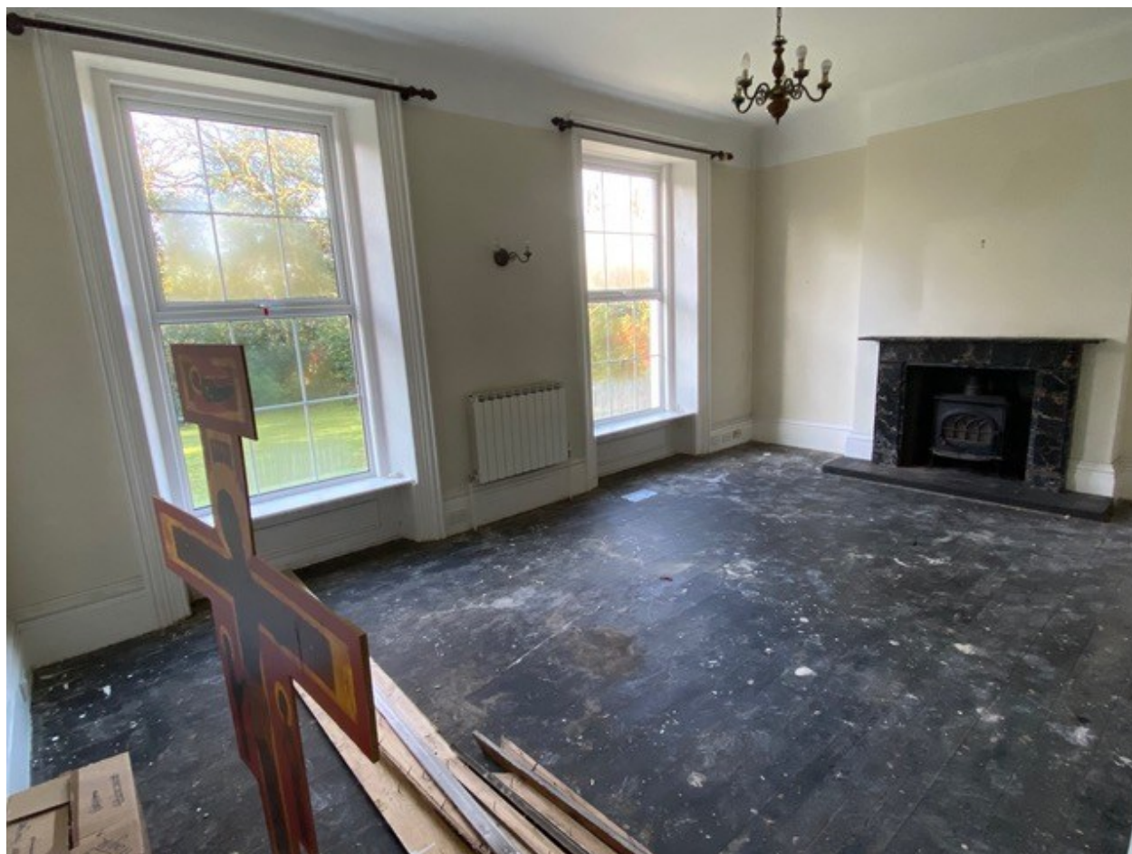
Reception room waiting for refurbishment
