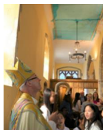
The Archbishop inspects the ceiling in 2017.
