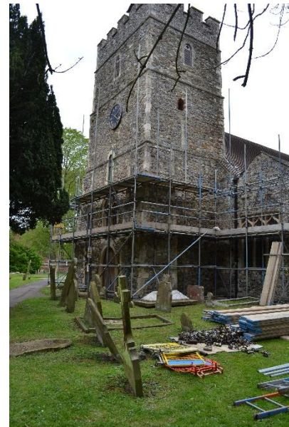
Major Building Works at Sturry
